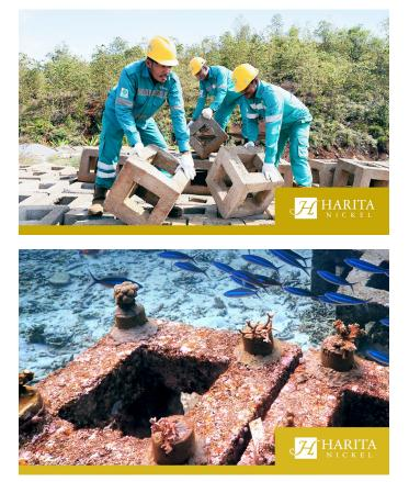
Trimegah Bangun Persada converts its nickel slag into bricks and artificial reef structures
