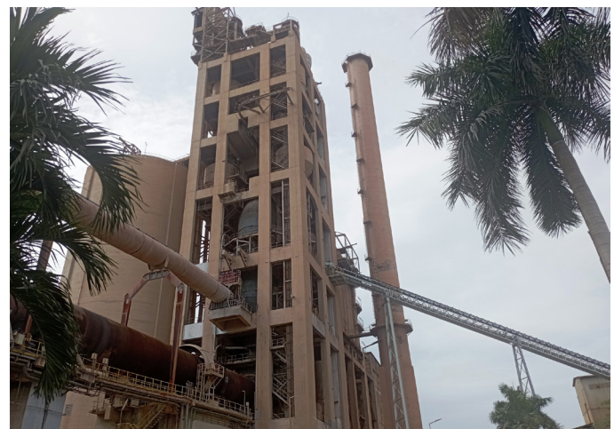
New kiln system in operation
