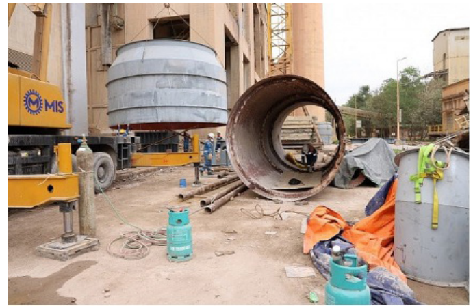
Construction of new kiln system
