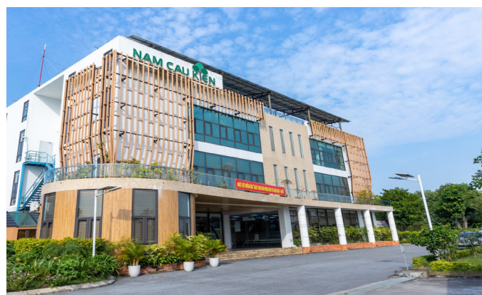
Solar power for office building at Nam Cau Kien IP
