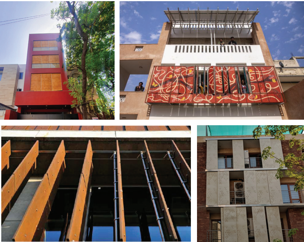
FIGURE 35: EXAMPLES OF EXTERNAL MOVABLE SHADING (EMSYS)
