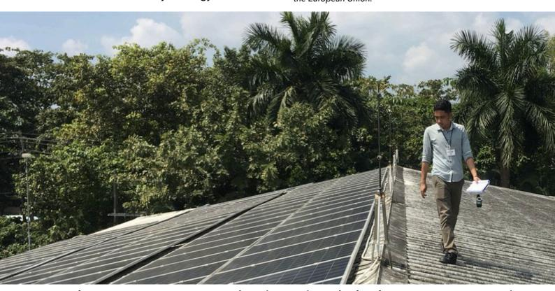
An engineer from SMART Myanmar inspects the solar panels on the first factory in Myanmar to implement rooftop solar, a garment manufacturer in Yangon. Since this factory's 80 kW system was installed another five garment factories have also implemented solar PV. The largest of these systems has a rated peak generation capacity of 250 kW.
