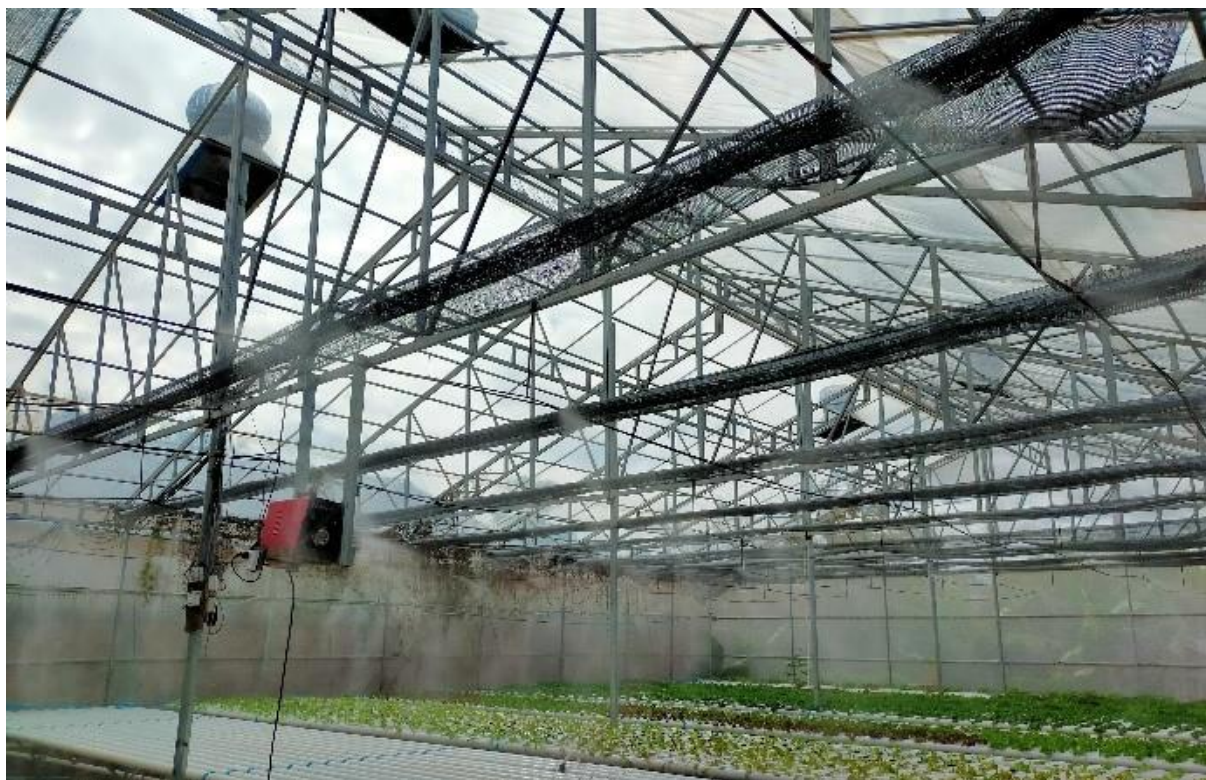
Figure 2: Misting machines in operation inside a net house
