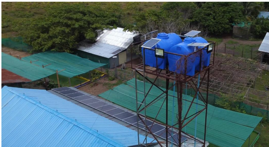
Figure 17: Elevated Water Tanks with Solar Panels
