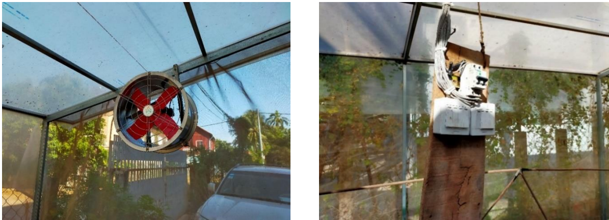
Figure 3: Cooling system in the nursery – exhaust fan and the switchboard with breakers.
