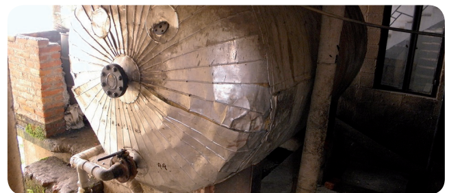
Improving an insulation for more efficiency
