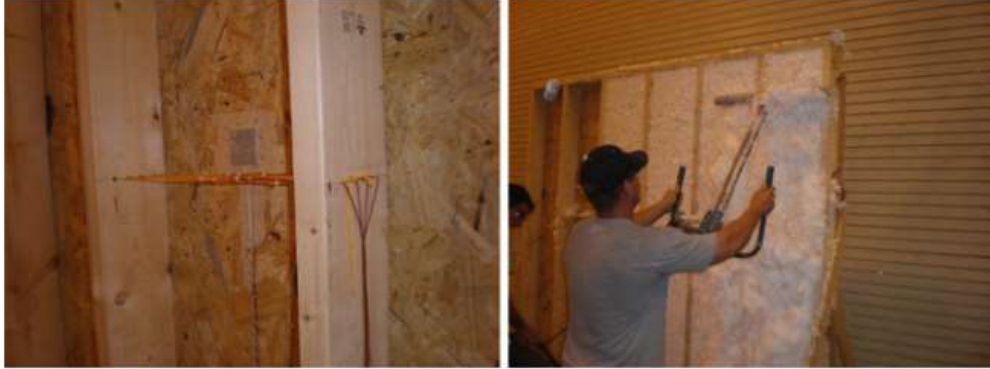
Figure 34: Installation of the test wall containing PCM-enhanced fibreglass insulation. (Kośny, 2015, p.37)
