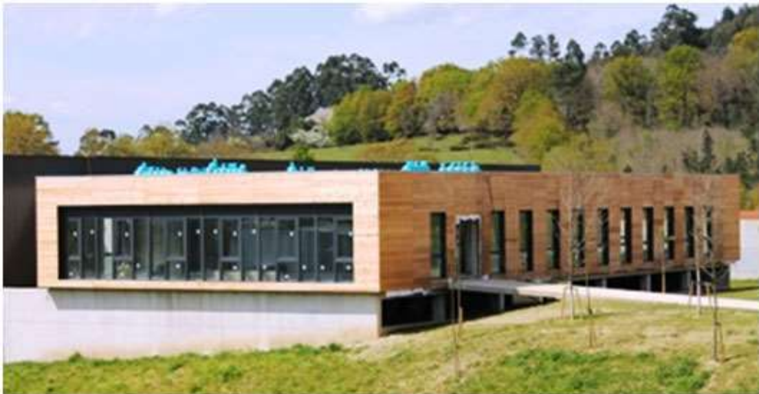
Figure 37: Demonstration building from B-first programme. (BFIRST-FP7)
