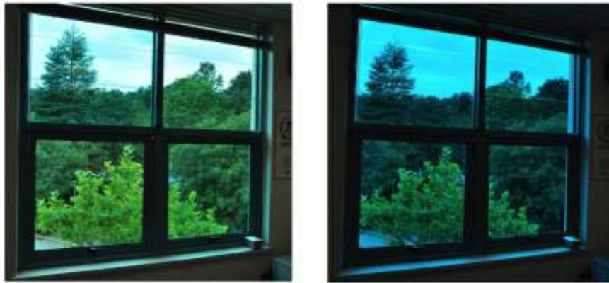
Figure 28: Example of a smart glass technology. Right:less transparent , left: more transparent (Albright, p.17)
