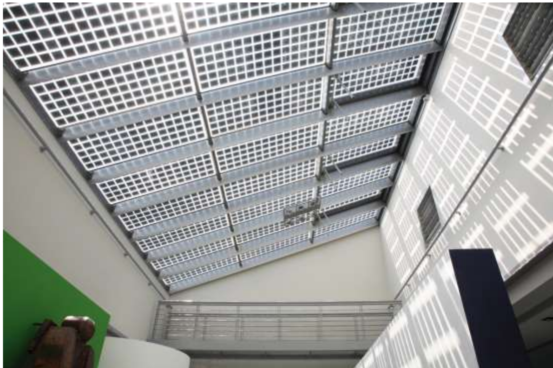
Figure 38: Example of transparent PV glass application. (Sapa Solar)
