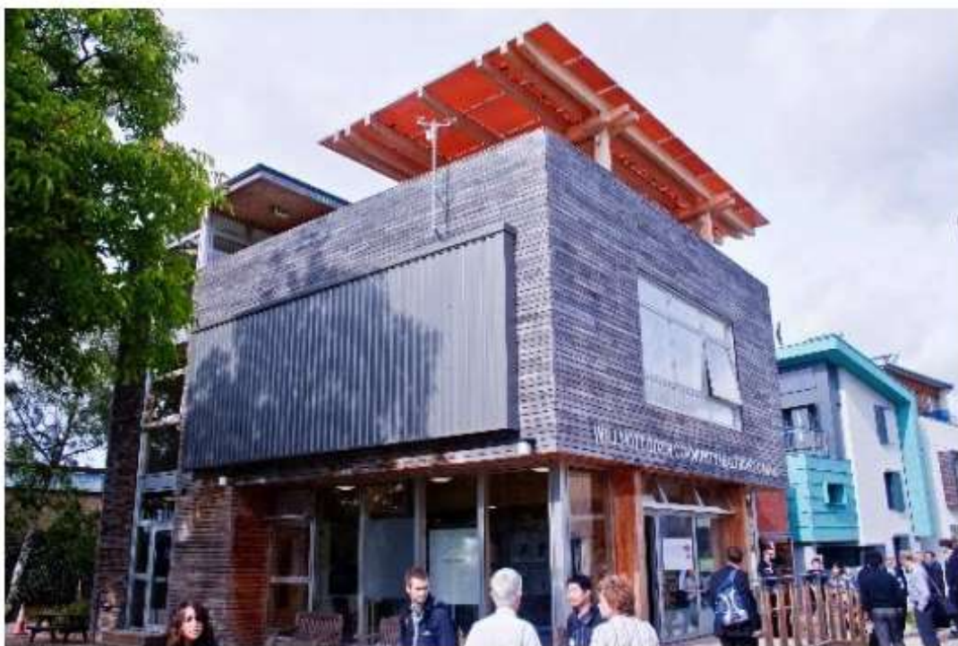
Figure 36: Example of BIPV, PV panels as canopies. (Polysolar Limited, 2015, p.19)
