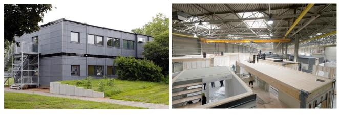
Figure 10: Energy Efficient pre-fabricated wooden containers in Germany
