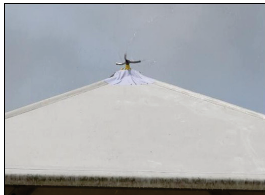
After: Installed water sprinkler and insulation at the roof
