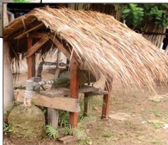
After: Installed roof shade to protect the motor from direct sunshine
