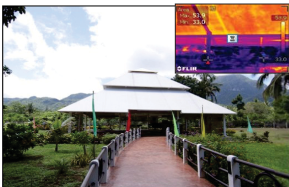
Before: No cooling system at the roof. The heat of the sun directly hits the tent (conference pavilion) roof and radiant heat reaches 53.9 °C inside.
