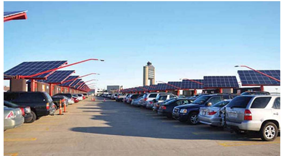
Solar 'trees' installed on the garage, Boston Logan International Airport, USA
