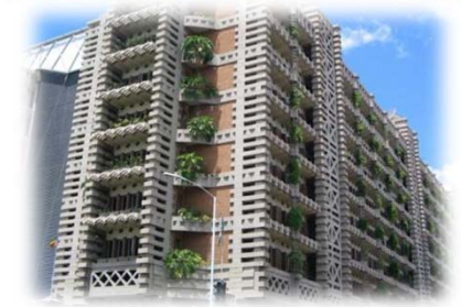
Eastgate: Sustainable building in Harare.
