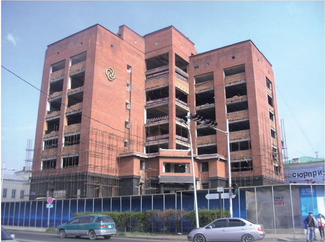
Figure 16 Demolition of the 10-storey building in UB
