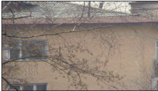
C. Asbestos roof of an apartment building
