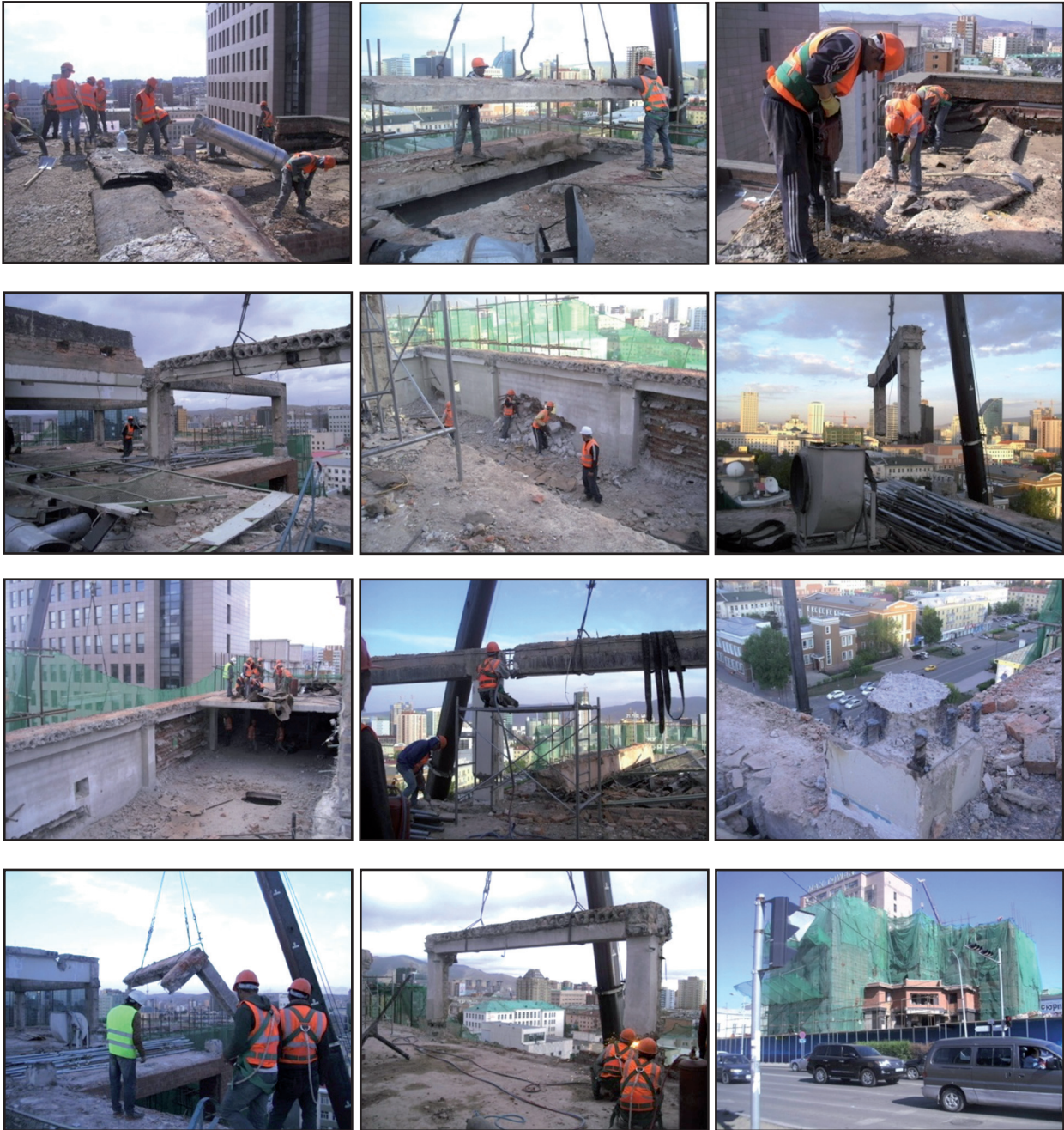
Figure 17 Different stages of the demolition process
