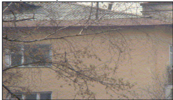
C. Asbestos roof of an apartment building
