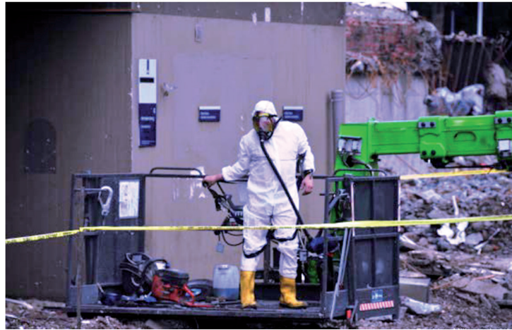
Figure 24 Asbestos sanitation in Netherlands
